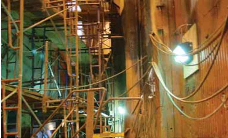
Wall packs come in High Pressure Sodium and Metal Halide from 50 watts to 400 watts.
