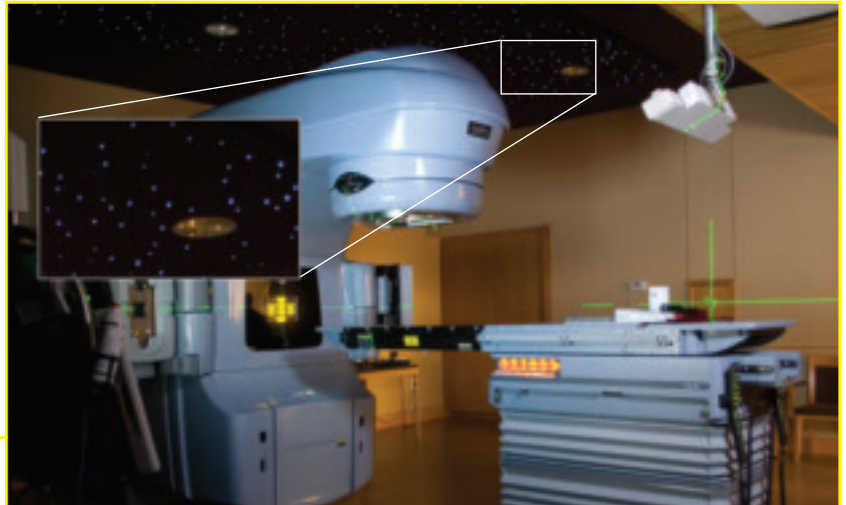
The linear accelerator room where patients receive radiation treatment has unique star field ceiling lighting to help patients relax. Recessed fixtures with dimmable CFLs (compact fluorescent lights) provide brighter lighting when needed. The control panel for the accelerator also includes controls for the room lighting.
