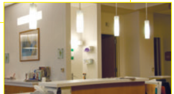
Mini pendants using CFLs add a decorative touch at the nurses' station in the oncology treatment area and they provide good lighting for the counter and area tasks.
