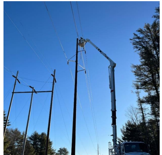
Figure 24. Replacement of Wooden Poles with Steel Poles Along Section 80 Transmission Line
