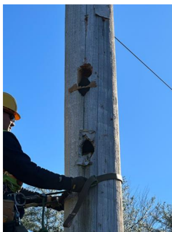
Figure 34 CMP Line Worker Inspecting a Wooden Pole
