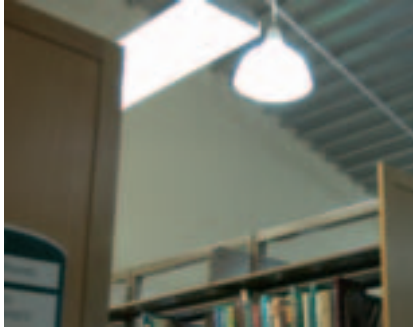
Large metal halide pendants provide good illumination for stacks with high shelves. These lamps provide a bright white light and the fixtures add to the decor.
